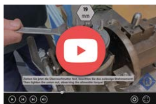
Tutorial 4CT cable installation
