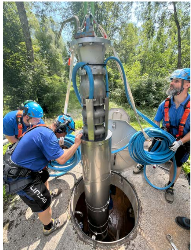
Installation at a depth of 30 metres in a drinking water well
