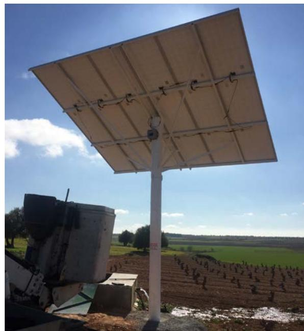
The frequency inverter can be installed directly on the mast, as it is optimally protected against environmental influences by its IP65 housing.
