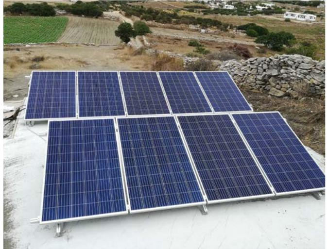
The system is powered by nine solar panels (standard polycrystalline 270 Wmp).
