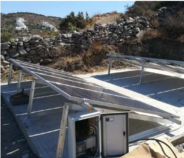
The Drive-Tech MINI Solar 2.015 MP frequency converter used is factory-equipped with Bluetooth 4.0 connectivity and can be controlled remotely via the mobile app.
